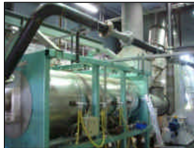
8 MW oxy-burner design for Lacq boiler
